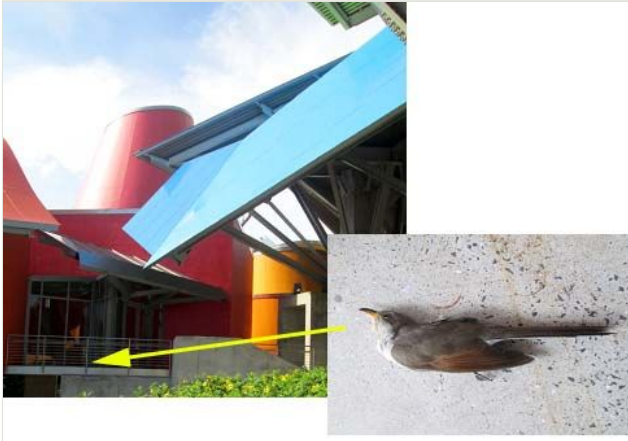
Figure 8. Some birds hit the glass of the Gehry's temporary exhibition corner during their migratory season.
